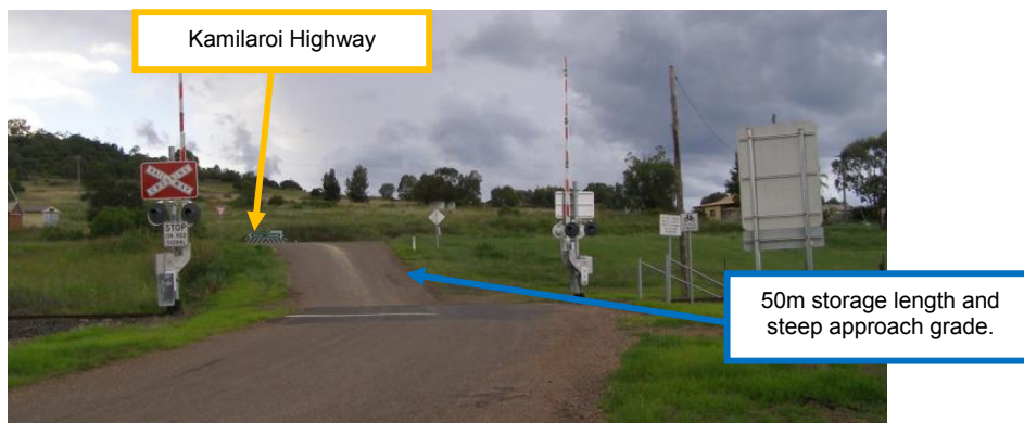
Figure 6-3 The short storage length and short-stacking risk at the Hogarth Street railway level crossing (photo is facing west).
