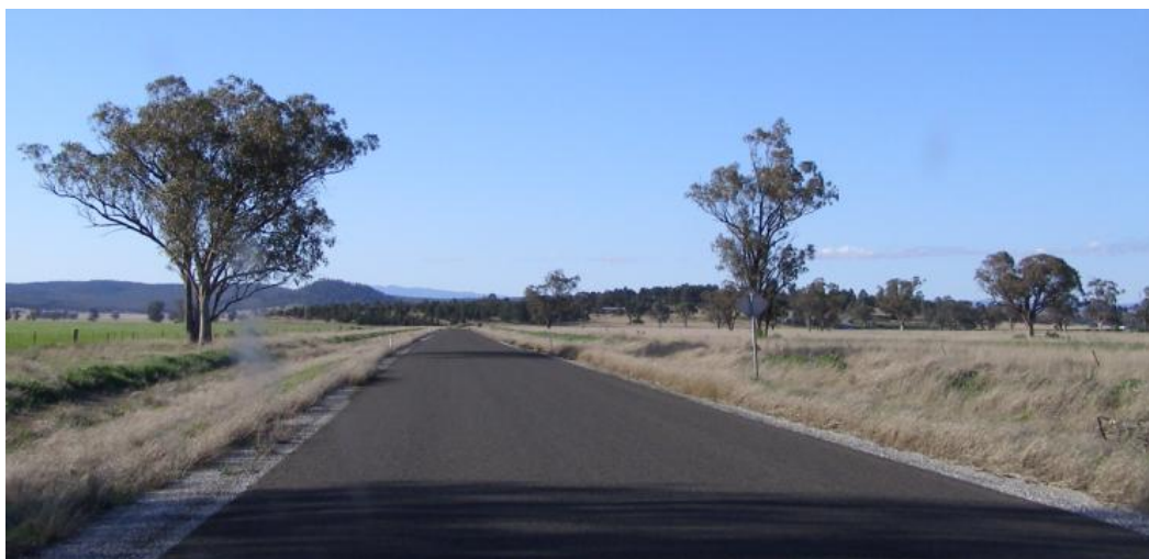
Figure 2-8 Leard Forest Road, sealed section between Manilla Road and Leard State Forest.
