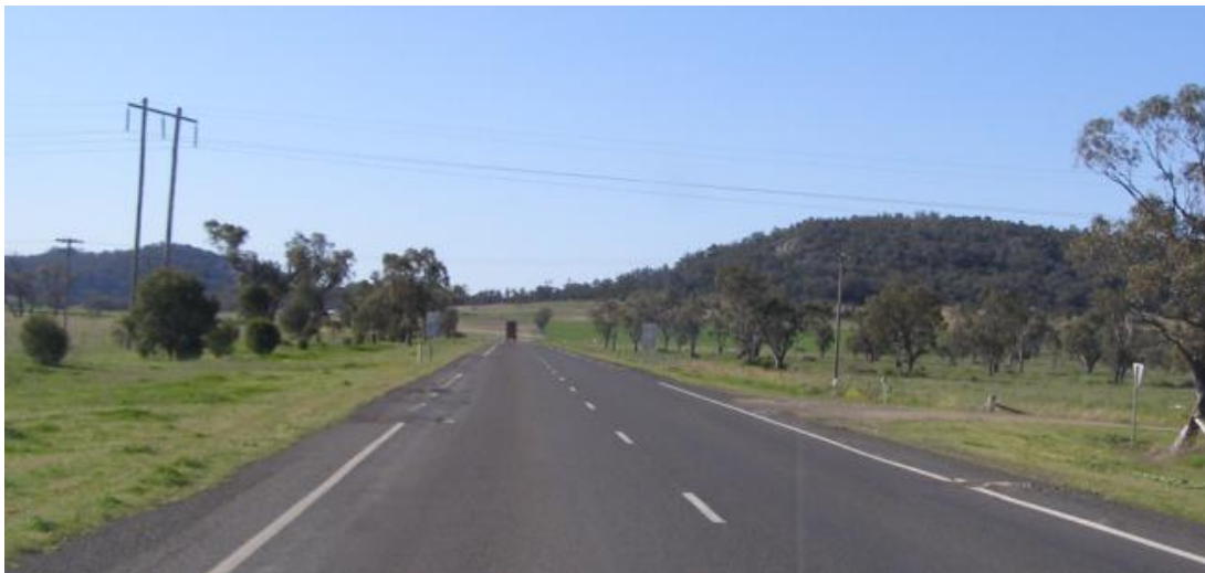
Figure 2-1 Kamilaroi Highway, looking northbound (the Manilla Road intersection is on the other side of the hill on the right-hand side of the photo).
