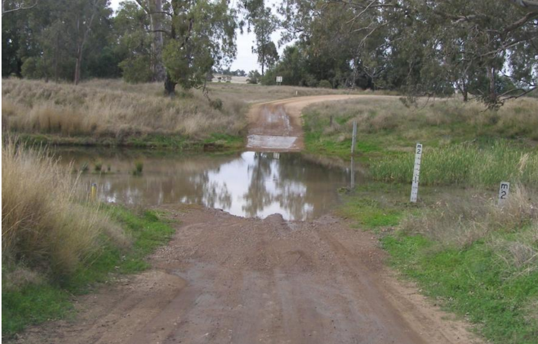
Figure 2-6 Therribri Road causeway at Maules Creek.
