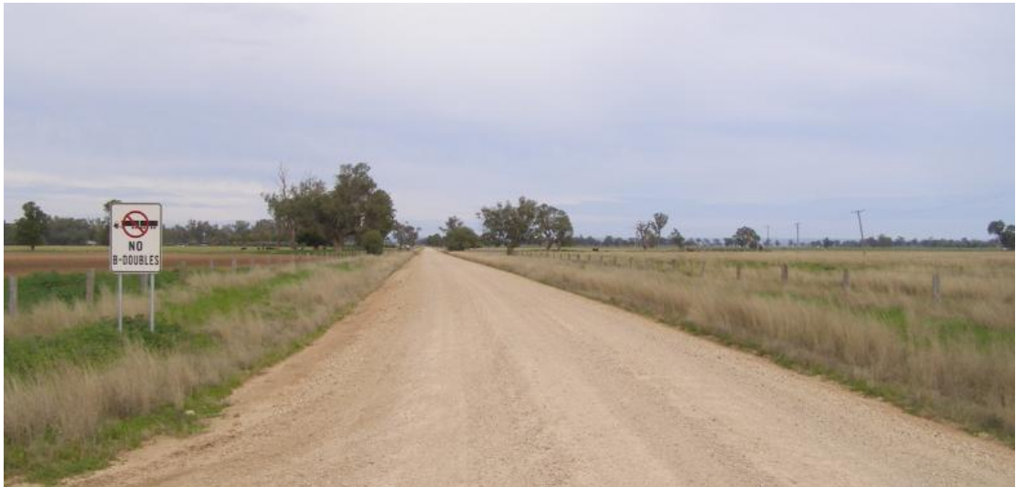
Figure 2-11 Harparary Road, looking west from Therribri Road.
