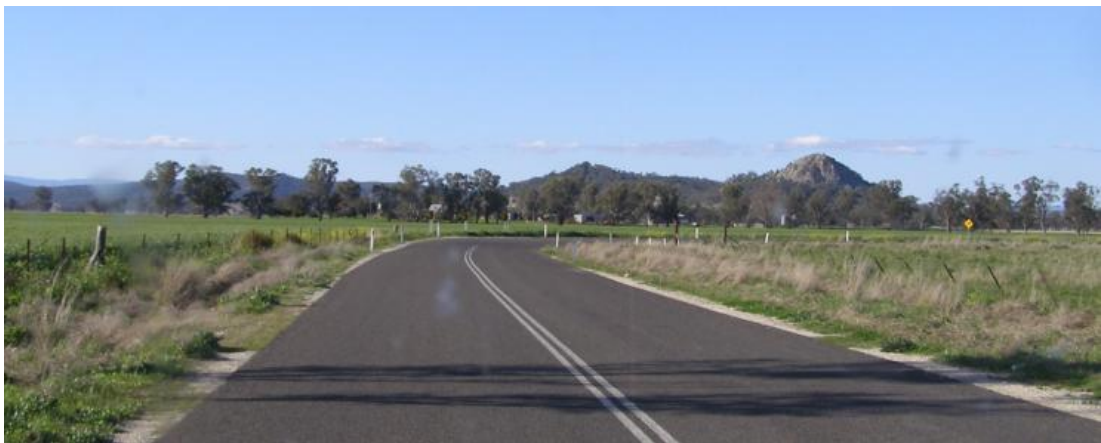
Figure 2-2 Manilla Road, looking eastbound at horizontal curve (Leard State Forest in background).
