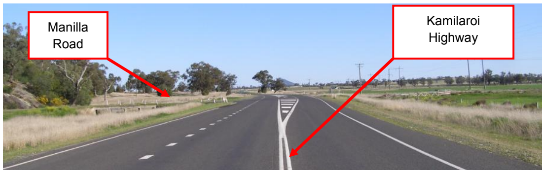
Figure 2-12 The Kamilaroi Highway/ Manilla Road intersection (looking south).
