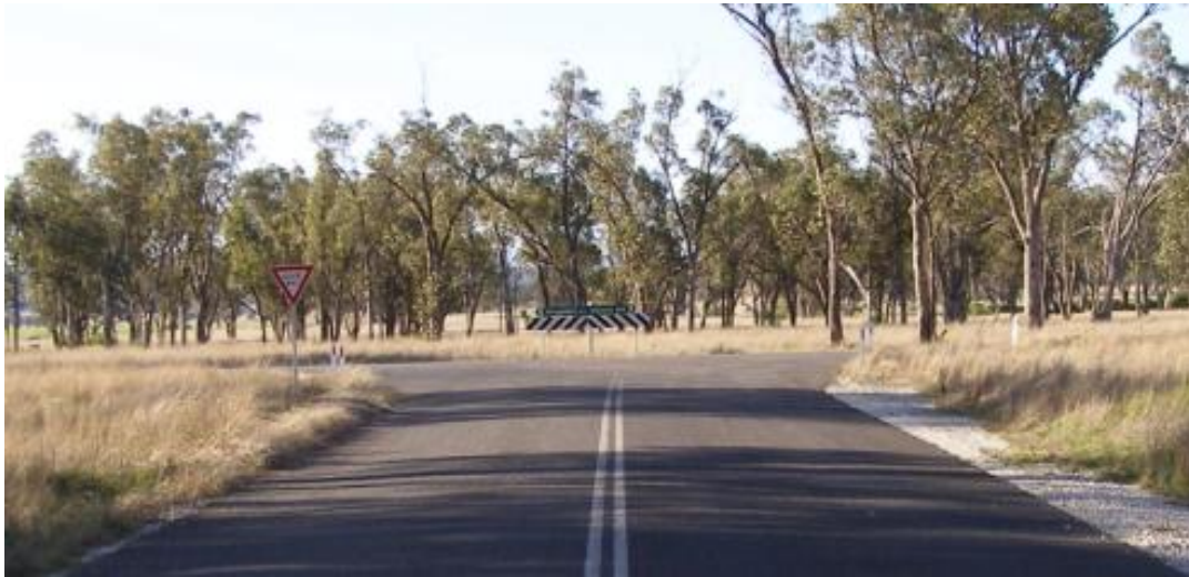
Figure 2-15 Barbers Lagoon Road looking north towards Manilla Road.
