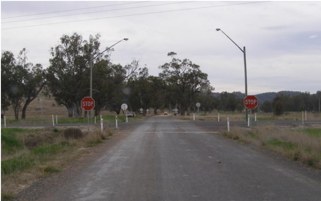
Figure 2-7 Therribri Road looking south towards intersection with Boggabri Coal haulage road.
