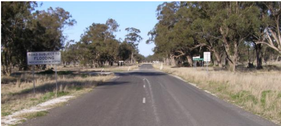
Figure 2-14 Manilla Road looking east towards Leard Forest Road (left).
