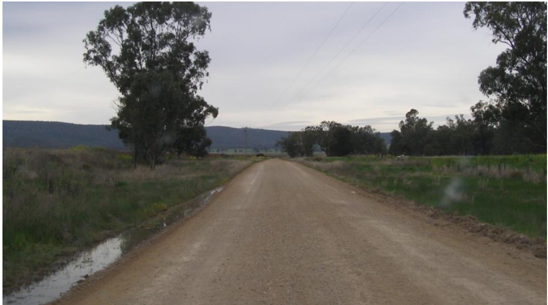
Figure 2-5 Water ponding at the road side due to a road side embankment.
